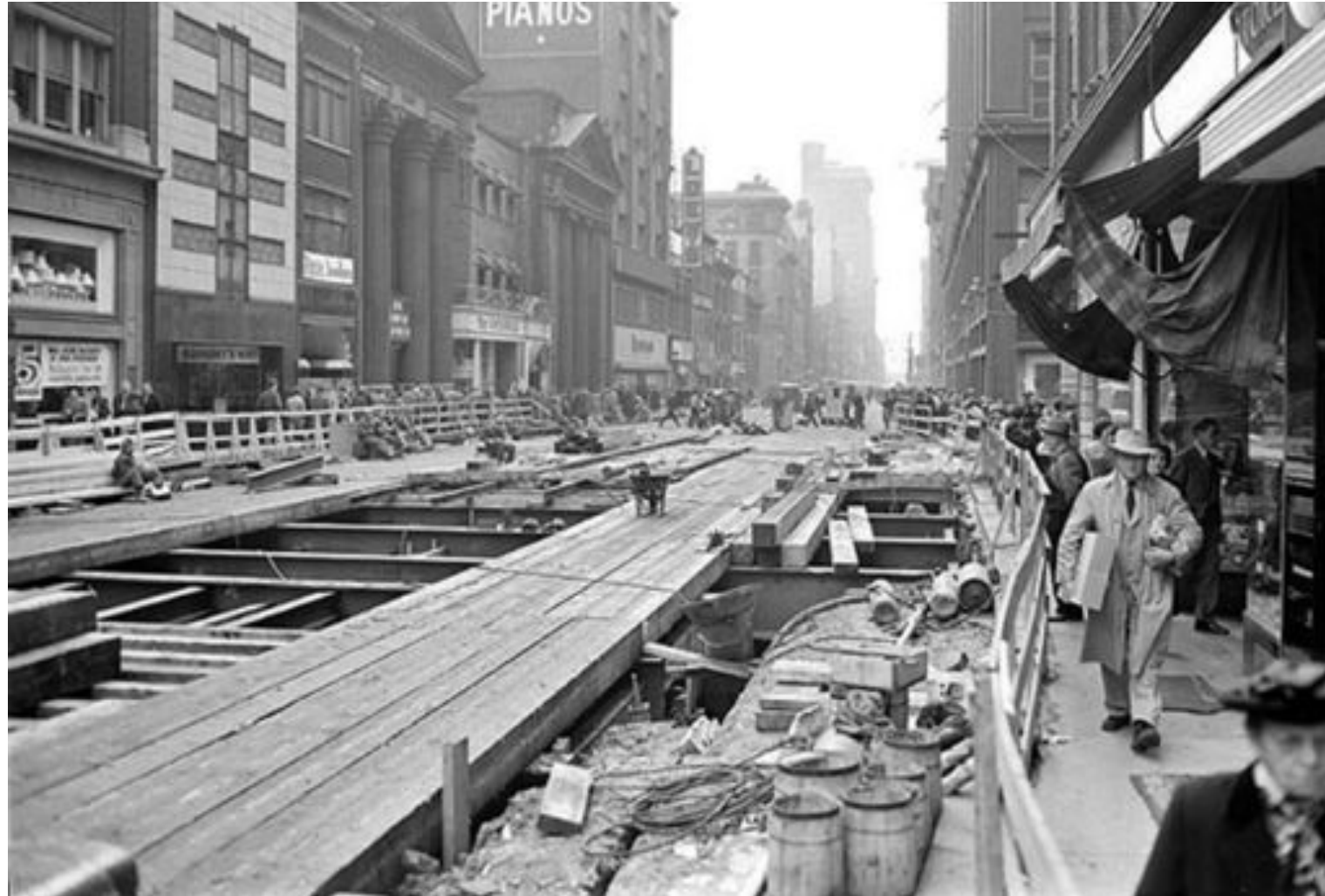
1 Yonge subway line construction, circa 1950
