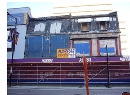
3 Sam's - during demolition
