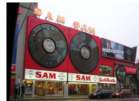
2 Sam's - before demolition
