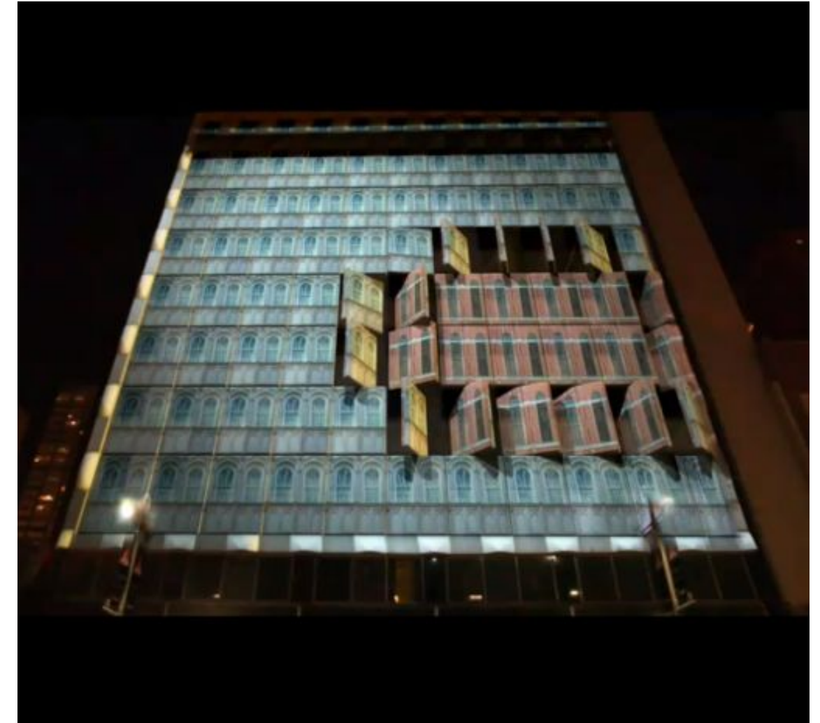
3 Digital media installation, Dallas
